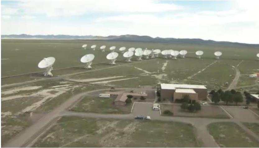
Each disk is massive, weighing 220 tons and is 82 feet in diameter and 94 feet high. It can rotate and tilt so as to aim in any given direction. Any disk can be moved along special railroad tracks. Since each disk presents such a large surface, they are subject to damage in high winds. In this event, the disk is parked pointing upward to present the least surface for the wind.
